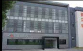
Holmatro Chine Suzhou, Province de Jiangsu, Chine Ventes et service
